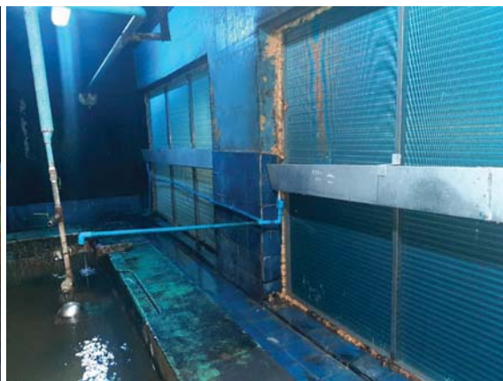
Tray , PVC pipe connect fill to pit
